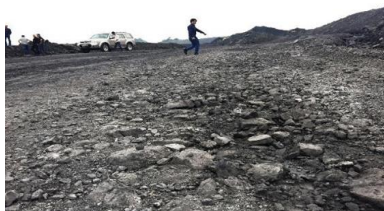
(b) Post mining rock material used for road construction
