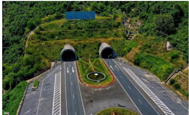
Figure 1. Deo Ca tunnel project.
