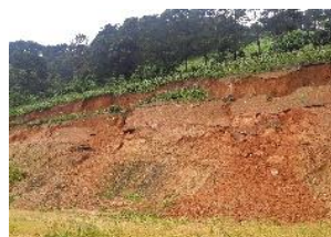
b. Soil rotational slide at MCC46
