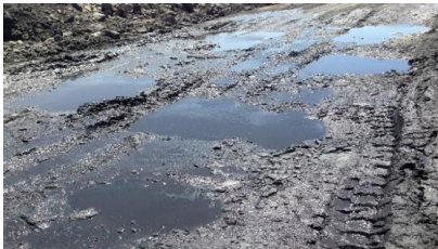
(a) Potholes formed on the haul road
