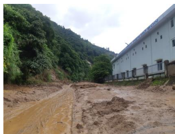
The control house of Hydraulic plant
