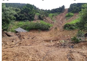
a. Soil flow at MCC14
