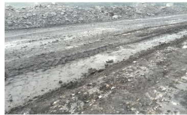
(a) Potholes formed on the haul road
